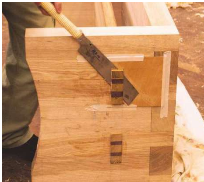
▲ Pic.7...and cut flush with a Japanese saw
